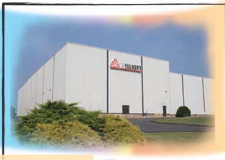
Exterior of the newly built test facility at the Mellon site
