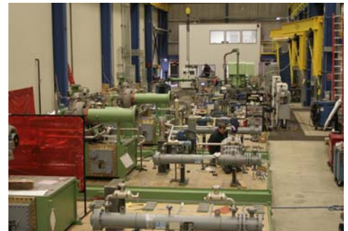
Three complete compressor units can be tested at the same time.
